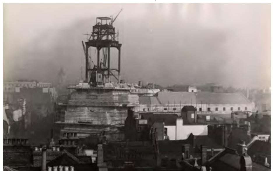
*The innovative Steel frame structure can clearly be seen.
